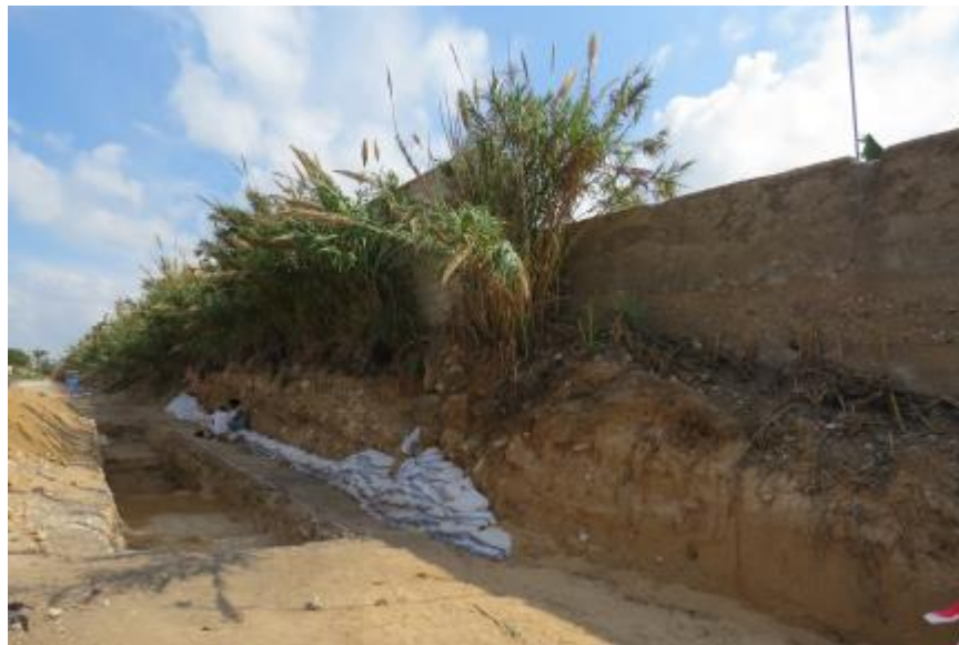
General view of the section and sounding trench.
