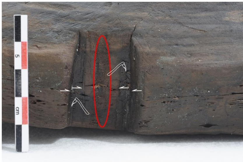
Fig. 7: Zambratija shipwreck. Detail of the limber hole of the floor timber R2 positioned east of the keel plank. (©A. Eeckman, 2017).
