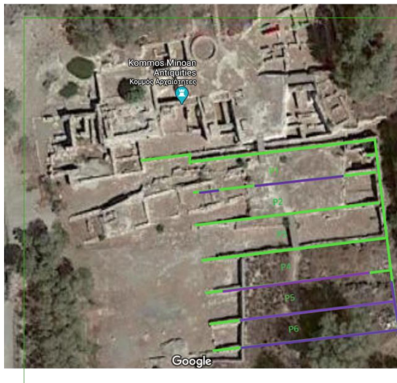
Fig. 14: Satellite photo of the harbour installations (Property of Google Maps, last access 04/02/2020). The plan of Building P is superimposed on the image to depict the excavated parts of the structure (in green) and their hypothetical continuation (in purple).
