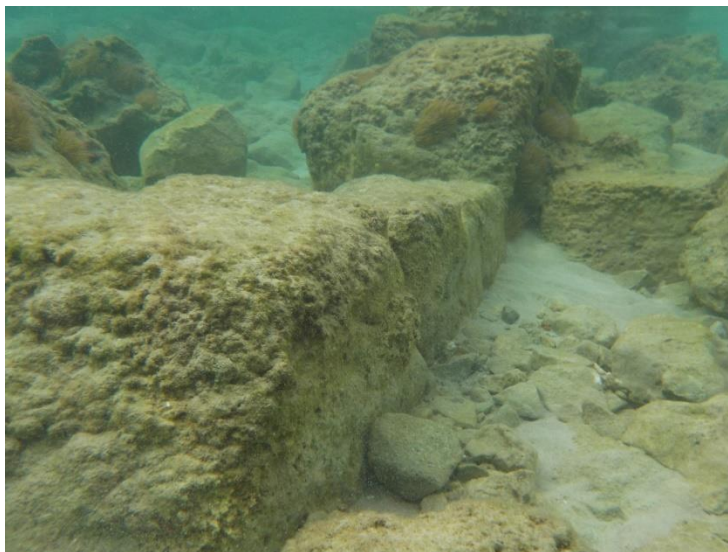
Fig. 11: Close up view of the end of the eastern wall, from the north to south (photograph by the author)
