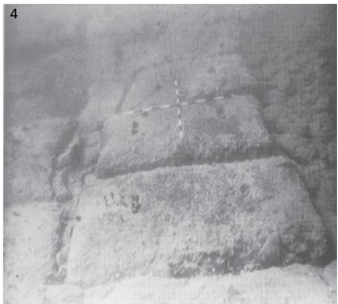
Figure 4. Photos of Zireh taken by Poidebard dating to 1951 show the maritime remains: 1: general view of old Sidon, 2: plan view of Zireh, 3: bollard, 4: jetty foundation
