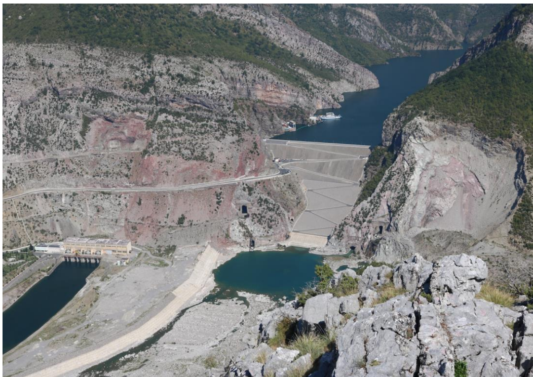
Fig. 6. Komani's dam, upstream of Shurdhah's Island (Courné, 2020).
